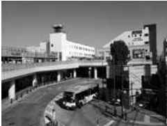
保谷駅南口 Hoya Station South Exit
